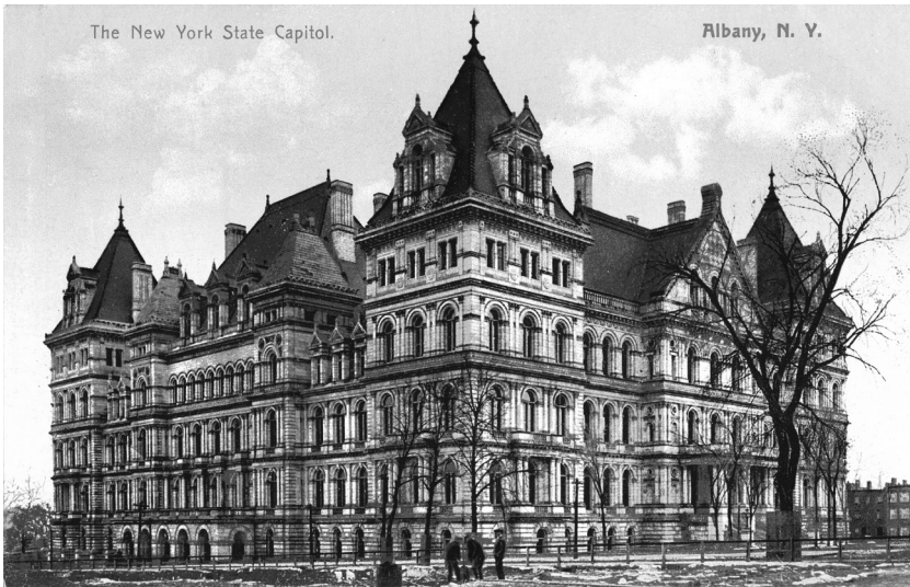
FIGURE 4. Bluestone quarried from land owned by Alfred Conyes's father and stone quarried by prisoners from Sing Sing Prison were used to build the State Capitol in Albany. Photo courtesy of the New York State Library.
