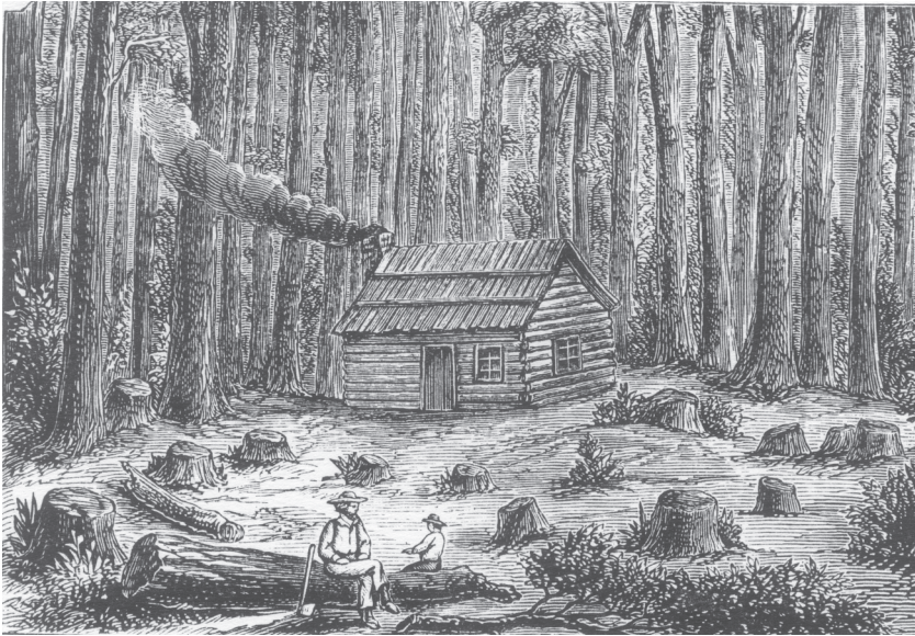
The McMaths home may have been like the Nowlin's first house, built in 1834.
