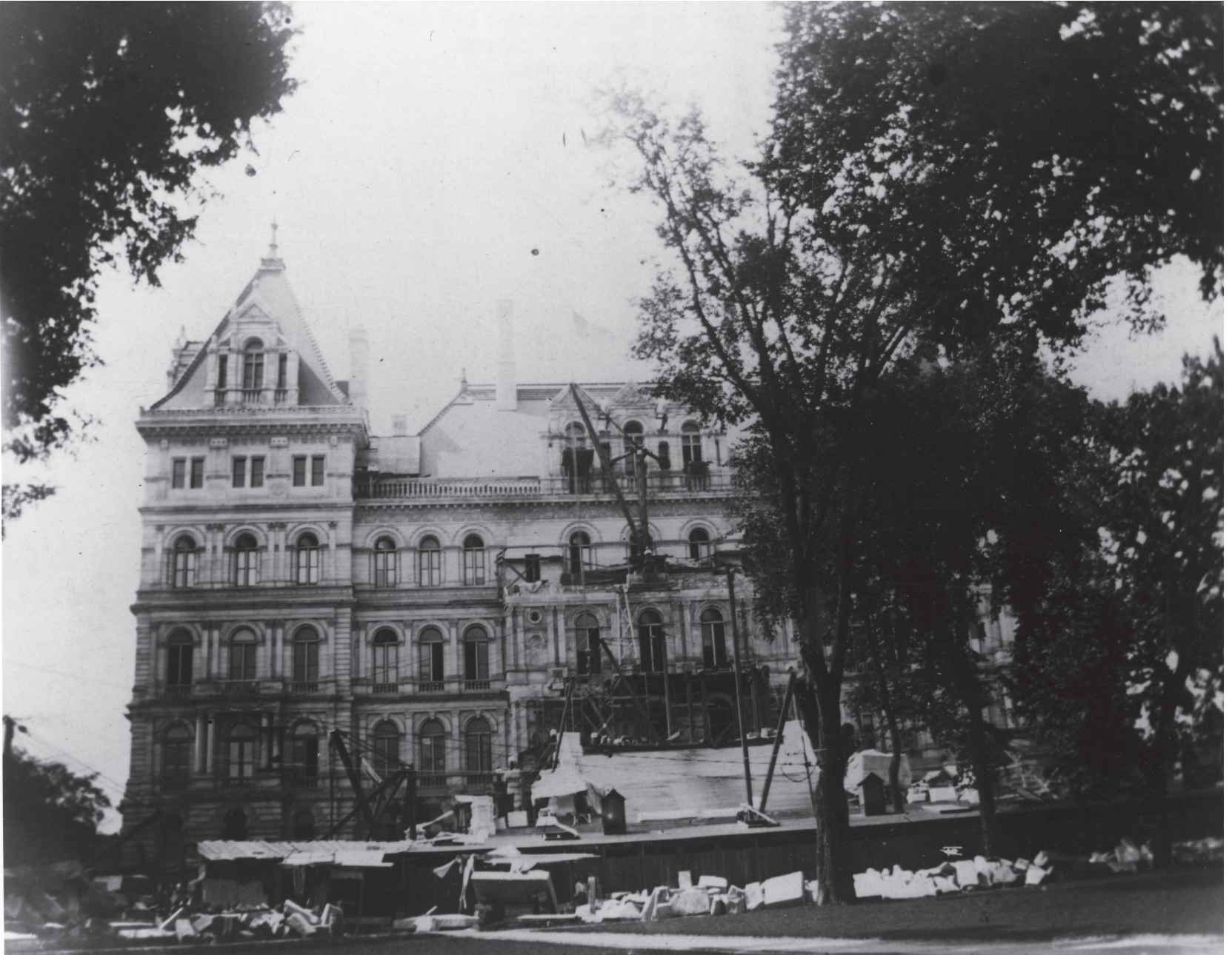
The east facade of the Capitol during the final phases of construction, looking up State Street, 1895
